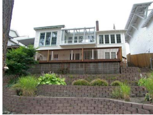
Home from the waterside. This backyard has been carefully terraced and contains many spaces to enjoy the water view, sun, peace and happiness.
