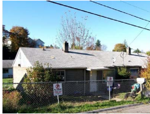
Left unit. Fenced back yard. Wood siding.
