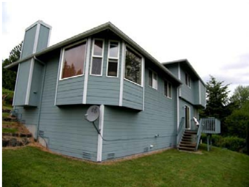
Back of home closest windows are to dining room facing south, then windows to kitchen and upstairs is master bedroom window. Glass slider is to the deck.
